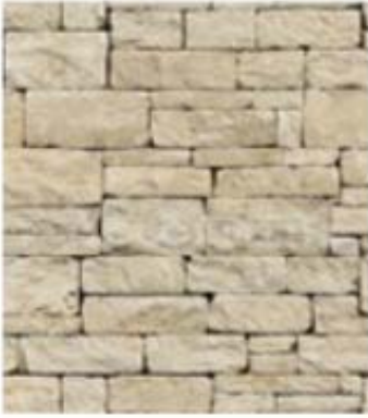
Stacked rectangles (un-grouted)
