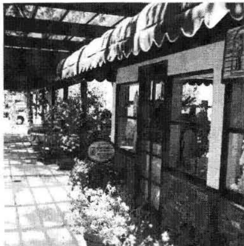
Door and Window Panes
